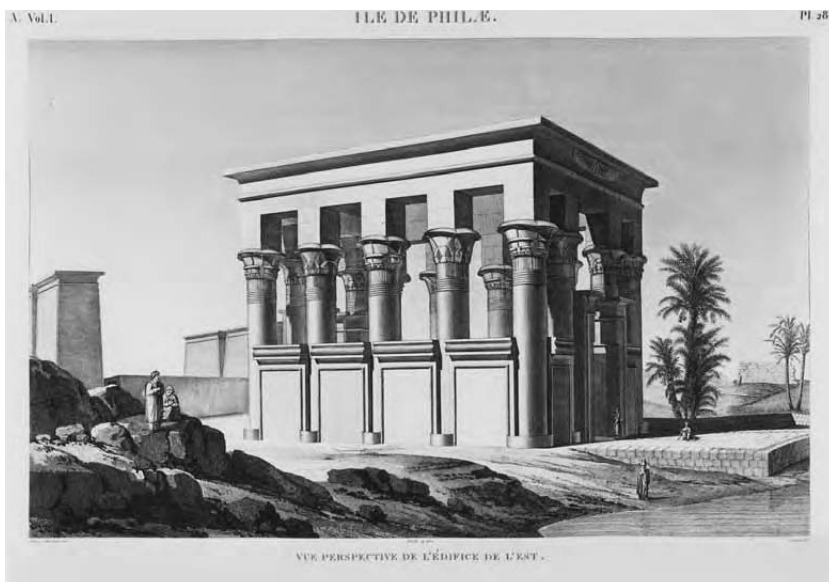
Plate 25 The so-called ‘Kiosk’ of Trajan, also known as ‘Pharaoh’s Bed’, on the Island of Philae, an essay in Romano-Egyptian architecture, begun under the Emperor Trajan (AD 98–117), and left unfinished. The capitals are of the papyrus type, and the spaces between the columns are filled to about half the height of the shafts with walls (plutei), a motif that was employed by many Neo-Classical architects (St George’s Hall, Liverpool [1839–54], by Harvey Lonsdale Elmes [1814–47], Charles Robert Cockerell [1788–1863], and Robert Rawlinson [1810–98], has plutei). The abaci above the capitals have become enlarged blocks, presumably intended to be carved with Hathor- or Isis-heads. On the left are the pylon-towers of the temple of Isis (From Description , A, Vol. 1, pl. 28, GB/SM).
